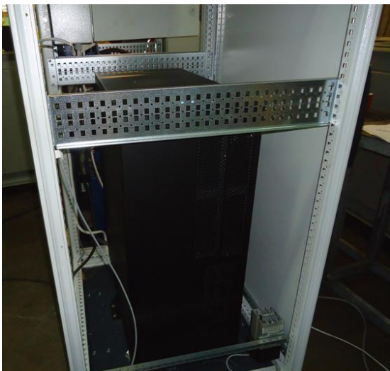
UPS / Unlimited Power Supply
